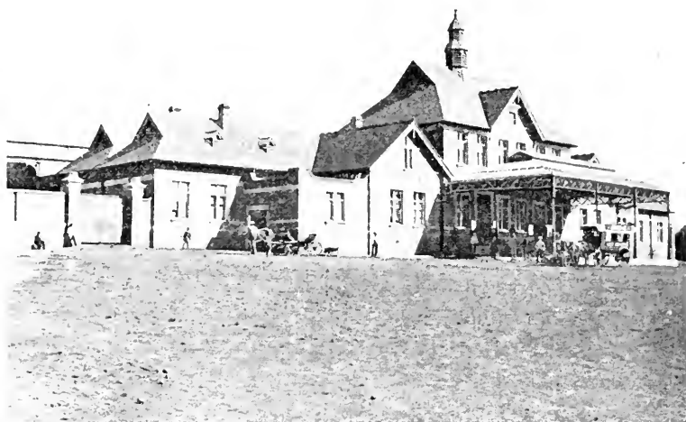
RAILWAY STATION, MARITZBURG.
